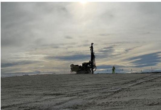
*Figura 6 Hincado*
