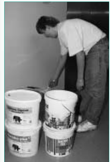
Natural paints used in Dunkerque, France
