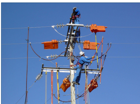
Fig. 16: Correction of intersection poles to eliminate the electrocution risk.
