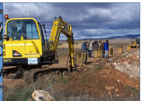
Fig. 18: Placing underground a high tension line in ZEPA "Laguna de Gallocañta".
