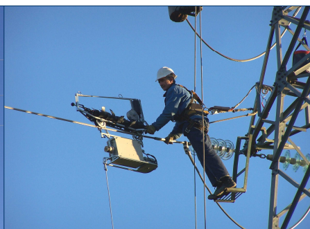
Fig. 17: Marking a conductor of a distribution line by guided robot.
