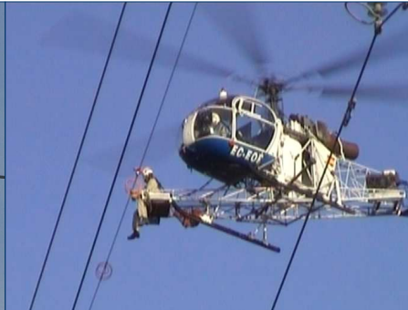
Fig. 14: Manual placement of markers by helicopter in the lines with tension.
