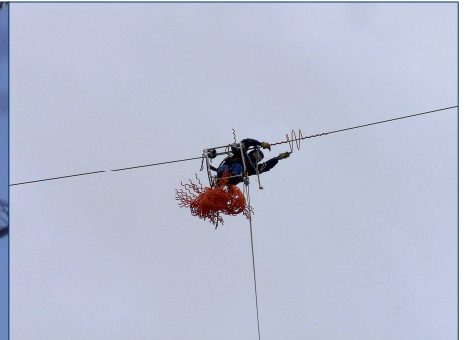
Fig. 15: Manual placement of markers by special device in line without tension.
